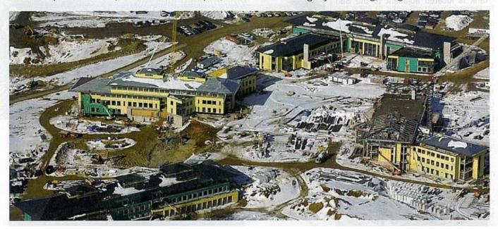
garage has approximately 600,000 sq ft for parking and each office building has an average of 100,000 sq ft of supported areas. A man-made brook will flow in the court-yard over the top of the parking garage.
